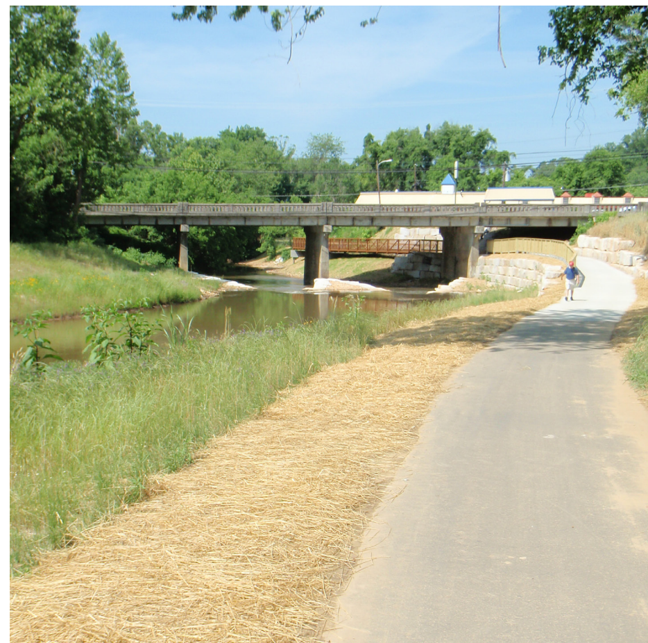
Ararat River Greenway and adjacent River restoration in Mount Airy, North Carolina
