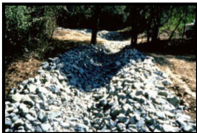
Drainage channel stabilized with riprap to prevent erosion
