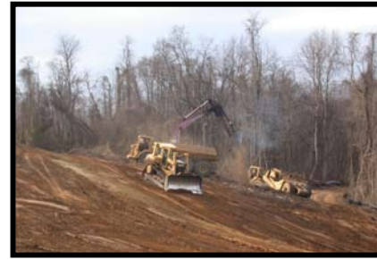
Construction sites can be significant sources of sediment to streams if proper ESC controls are not used
