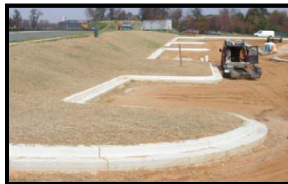
Hay applied to newly cleared area for immediate stabilization of soil
