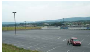
Excessive paving in parking lot
