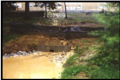
A muddy stream can indicate failing ESC practices upstream
