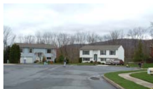
Typical 100-ft diameter cul-de-sac
