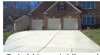
Typical driveway is fully paved
