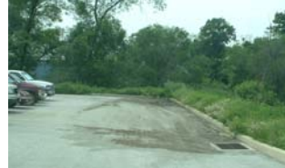
Parking lot runoff goes to storm sewer
