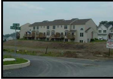
Runoff from this construction site in the Paxton Creek watershed has high sediment loads
