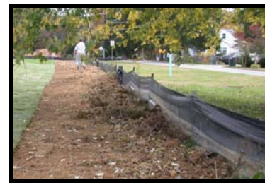
Perimeter control silt fence filters sediment from runoff leaving the site
