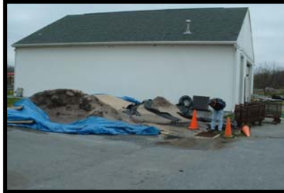
Inadequate cover allows pollutants to enter storm drain
