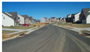
Typical excessively wide road
