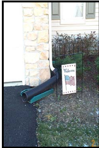
Rooftop runoff indirectly connected to stormdrain over driveway
