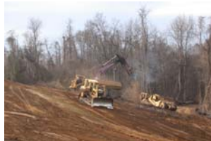
Typical site is mass cleared
