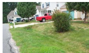
Vegetated open channel
